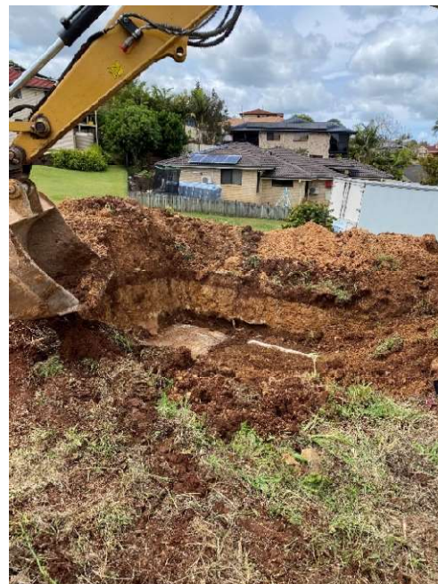
Photograph 2.2: Northern end of dip bath and dip pad exposed, with imported fill profile visible above.
