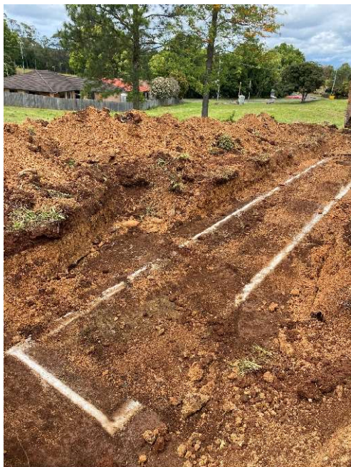
Plate 8.1: Top of the dip bath. The imported fill/cap profile is visible above.
