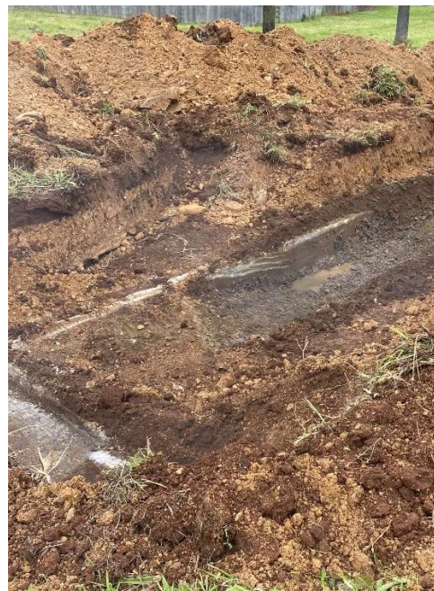
Plate 8.2: Northern end of dip bath showing exposed saturated gravel contents
